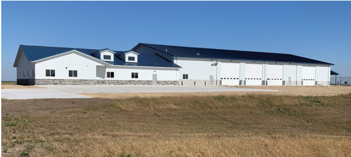
LPRW's new headquarters and main operational facilities.
