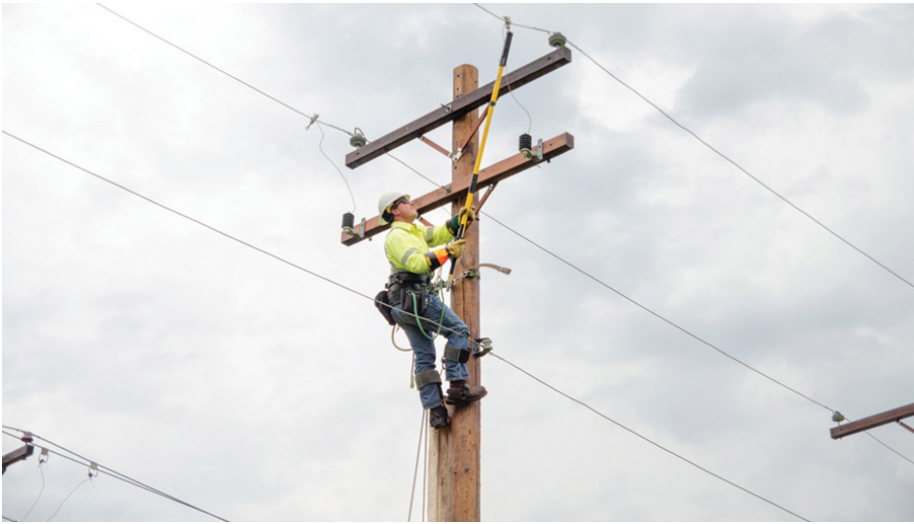
The arrester change-out event tested competitors’ ability to safely and efficiently replace a surge arrester—critical equipment that protects power systems from lightning strikes and voltage spikes. The task required technical precision, methodical work aloft on a utility pole, and strict adherence to safety protocols, all while racing the clock. The best time was accomplished by Landon Meier from Rochester Public Utilities, who completed the entire process in eight minutes and 44 seconds.
