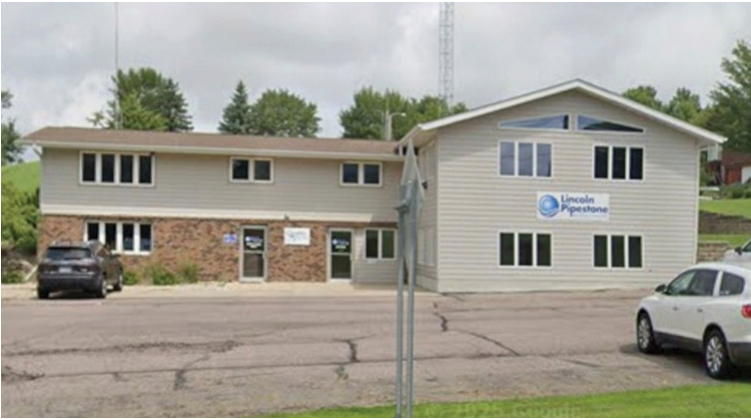
LPRW's old headquarters in a modified home at 415 East Benton Street in Lake Benton.
