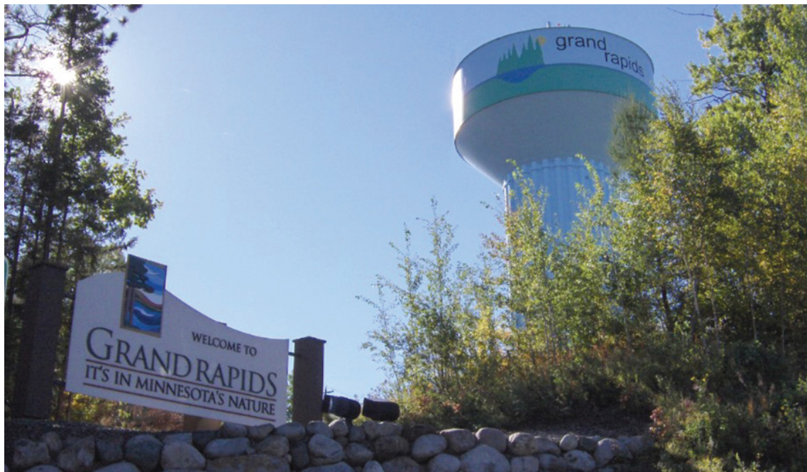
The water tower at the south end of Grand Rapids—long a beacon for residents and visitors—overlooks a community working to rebuild confidence in its water system and a utility strengthening its service by applying lessons learned from the 2023-24 Legionella outbreak.
