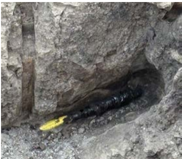
Digging exposed a leaking dresser fitting which had to be repaired to stop the gas leak. To the left, marks from a 26-pound frost bar used to determine depth are visible.
