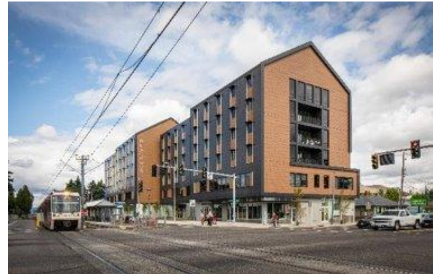
CCC's Blackburn Center opened in 2019 to provide all comprehensive services under one roof.
