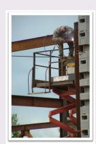
Platform access gate/chain must be closed & feet must be on platform. No standing on toeboard, platform rails, planks, buckets, boxes, etc.
