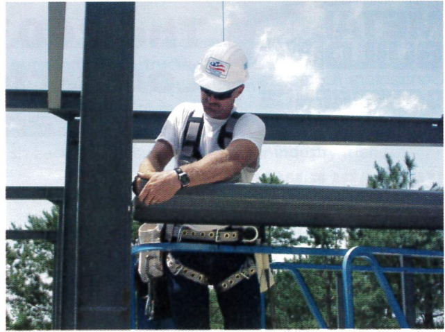
Keith Wood, Wil-Shar Steel Erectors was one of the "stars".
