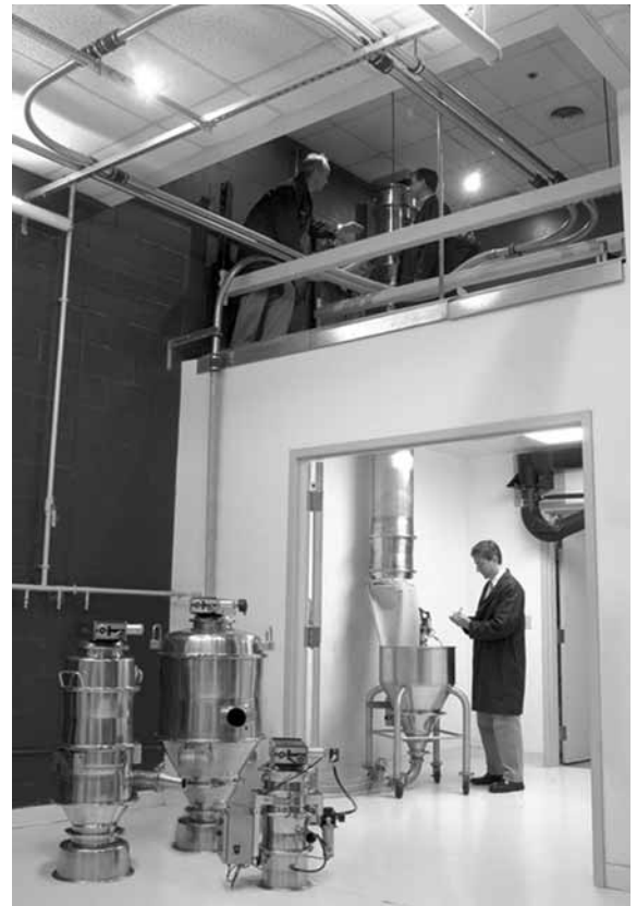
PIAB USA Inc.’s testing facility at its vacuum conveyor laboratory, Hingham, Massachusetts, allows customers to test the process in which they will move their powder, granule or fluid samples.
