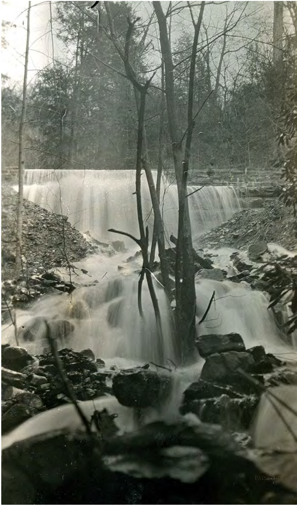
Historic Unnamed Spring Reservoir Below Dam ( https://pinemountainsettlement.net/ )
