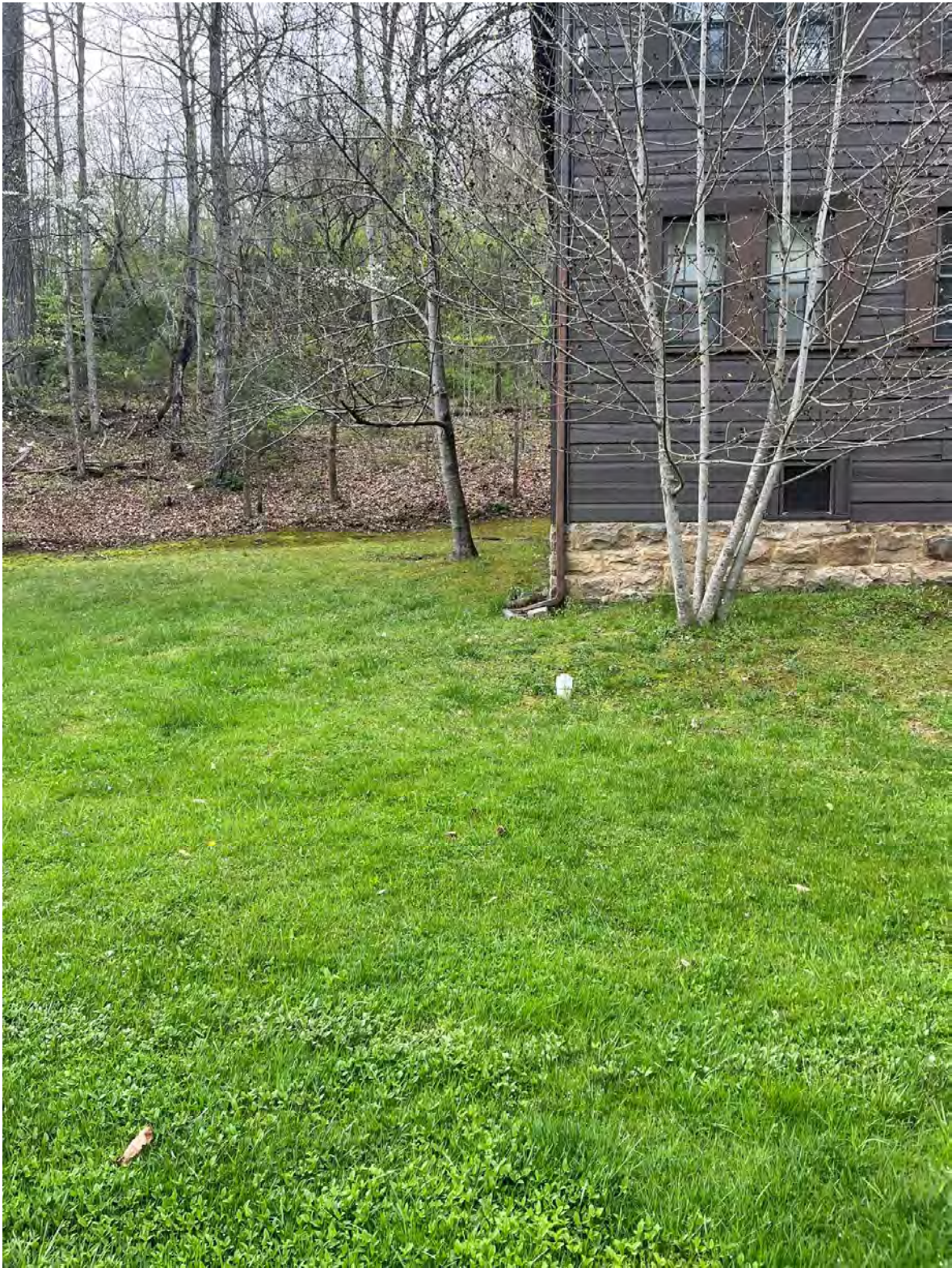
Septic System on campus of Pine Mountain Settlement School
