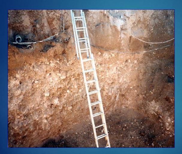
These two ladders which are lashed together are dangerous and not an adequate means of egress.
