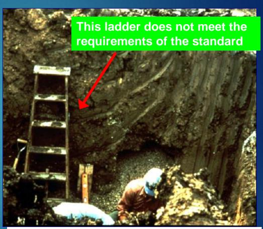
The ladder should extend 3 feet above the excavation
