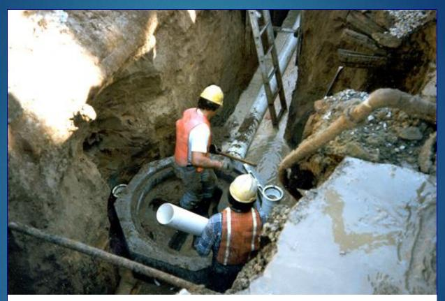
These workers must be protected from a cave-in. Note the water in the bottom of the trench. This is a very hazardous condition!
