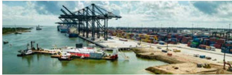
Project 11-Accelerating the Houston Ship Channel expansion for the economic and environmental benefit for the region. Port Houston and private industry are working together for today and future needs. To read more on Project 11 and updates, see page 4.
