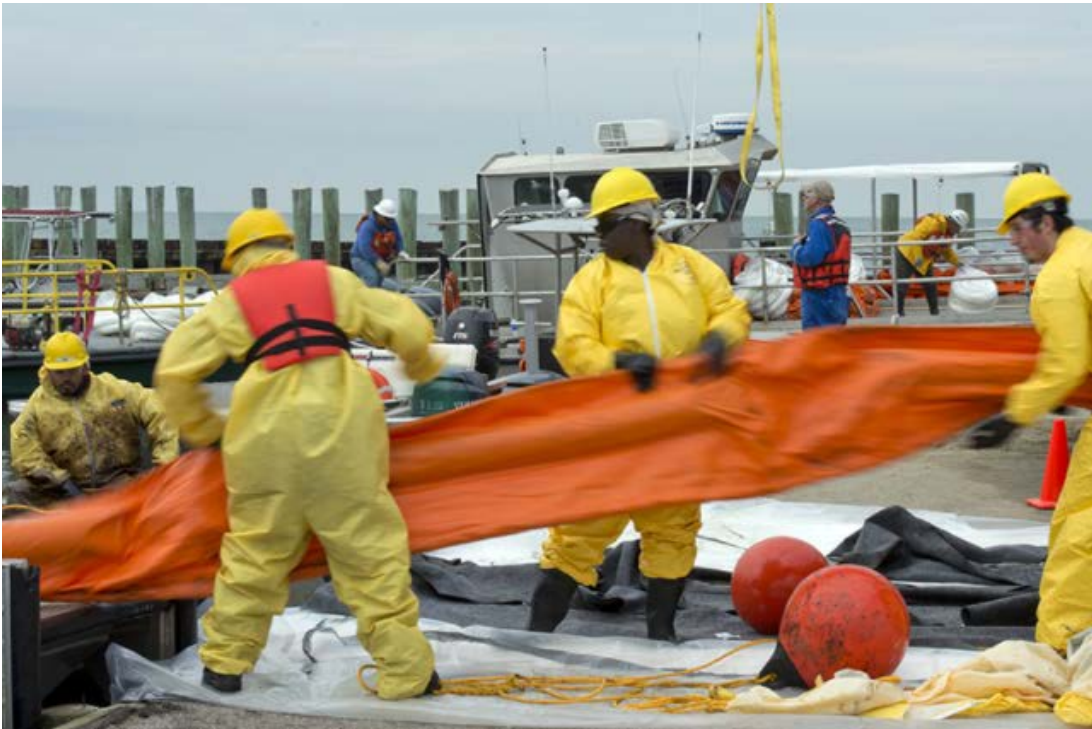
Workers deployed boom around the site of the oil spill in the Houston Ship Channel near the Texas City Dike. More than 71,000 feet of boom was deployed in response to the oil spill. Photo courtesy of the USCG.
