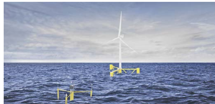
Ocergy’s OCG-Wind & OCG-Data platforms. Photo courtesy of Ocergy.
