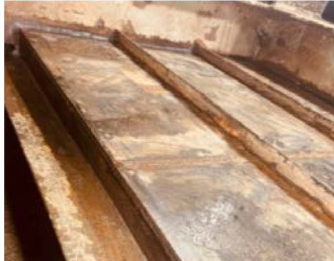
Figure 2: Post internal cofferdam built
