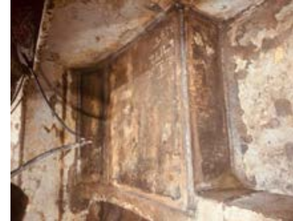
Figure 3: Forward internal cofferdam built around damaged area
