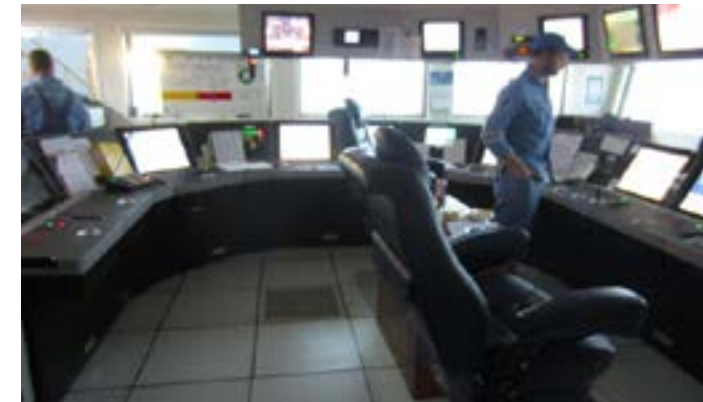
A fully digital bridge, linked to digital control and safety critical systems, and remote access.
