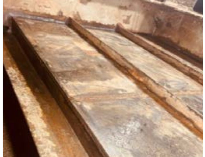
Figure 2: Post internal cofferdam built
