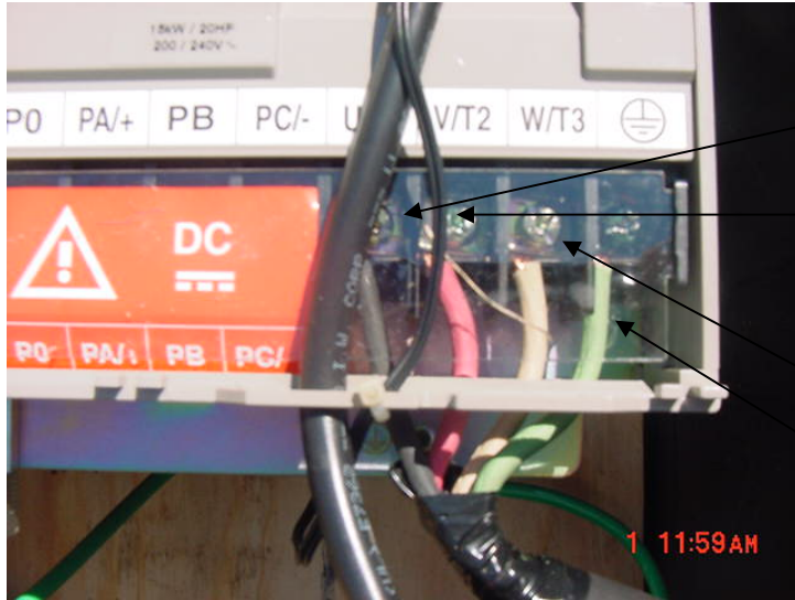
Figure D VFD Outgoing 240V Three Phase and External Grounding Connection
