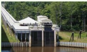
Water Intake, Distribution and Storage
