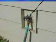
Device to prevent backflow from hose.
