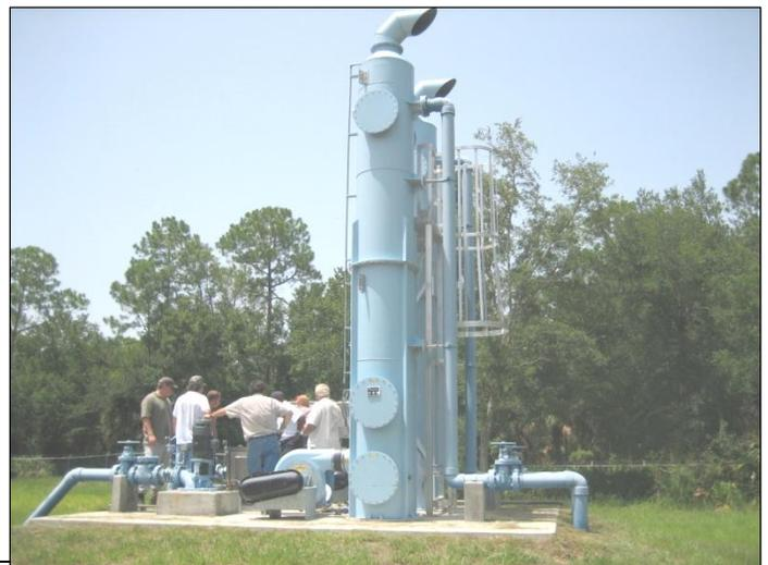
upward through the packing (countercurrent flow). The packing provides an extended surface area and impedes the flow of both fluids, extending the contact and to increase the gas-liquid interface. As water and air contact, VOCs and H<sub>2</sub>S, move from the water to the air. Iron, manganese, color, CO<sub>2</sub>, and organics are also reduced by oxidation in the packed tower.
