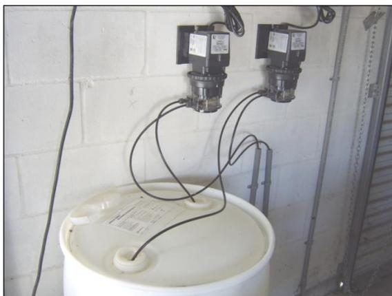
Phosphates are added to groundwater at the well head or at the pump intake before the water has a chance to come in contact with air or chlorine. This ensures that the iron and manganese stays in a soluble form. No sludge is generated in this method.
