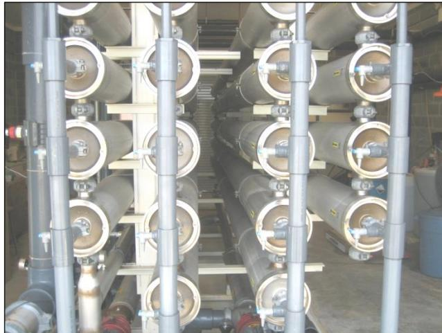
NF employs a spiral membrane configuration with larger pore size than RO, down to 0.001 micron. NF employs pressures between 100 to 200 psi for operation. Softening. 60-80% of all ions are rejected, 90-95% of divalent ions (sodium chloride) are removed, and organic compounds in the 300 to 1000 molecular weight range are eliminated, the technology is also very effective for removing color and DBP precursors.
