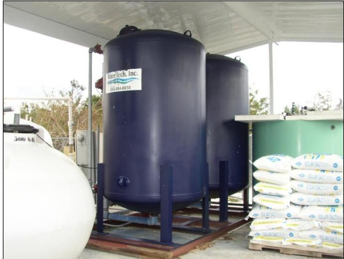
**Installed Costs: 3.** Very effective to remove DBP precursors, TOC, iron, manganese, arsenic, nitrates, uranium, color, odor, and taste. Sulfates, nitrates, and other ions compete for adsorption sites.
