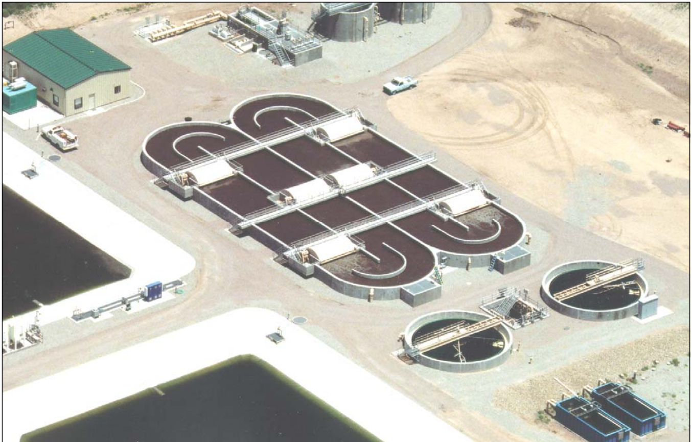
Figure 3 ~ Oxidation Ditches with Lakeside Aerators
