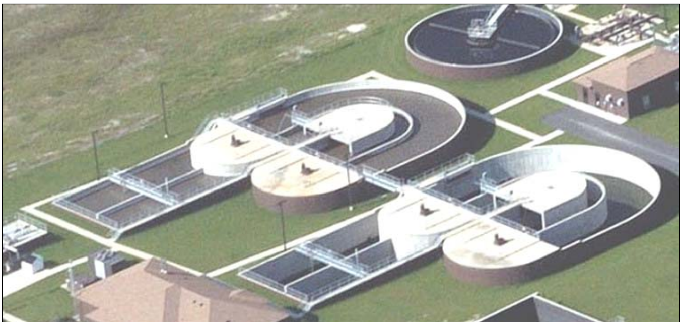
Figure 4 ~ Oxidation Ditches with EIMCO Aerators
