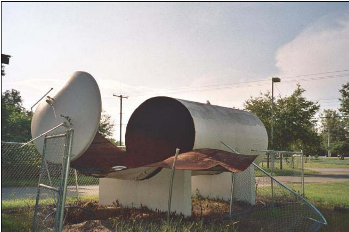
Hydropneumatic Tank Rupture
