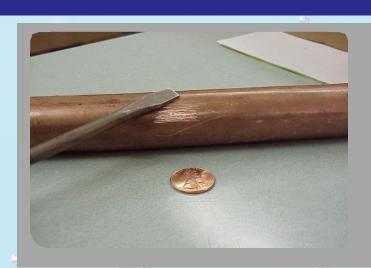
If the scraped area is copper in color, like a penny, your service line is copper. A magnet will not stick to a copper pipe.
