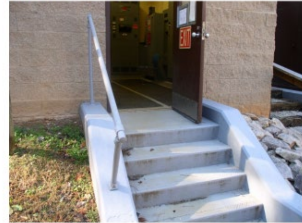
Figure 9 – Station with single flood door
