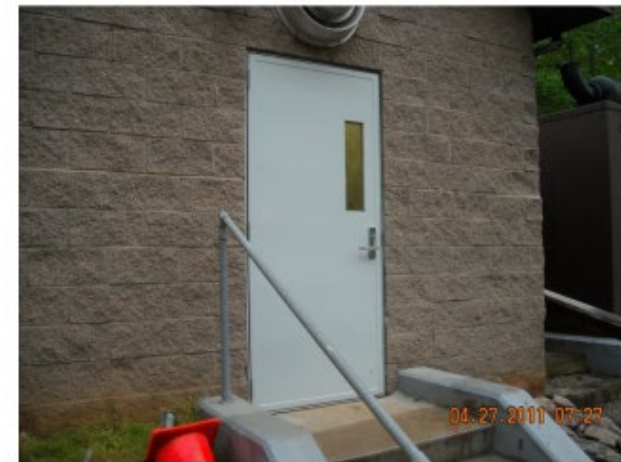
Figure 9 – Station with single flood door
