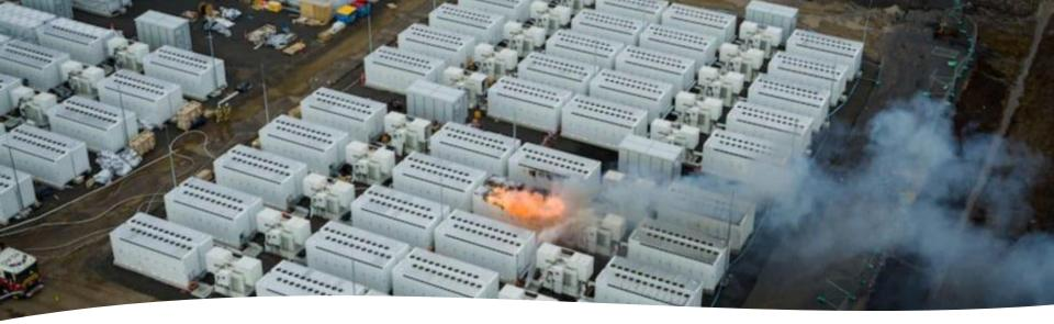
Lithium Ion Batteries Understand the risk - overcharging, overheating, cycling and aging Chemical composition - Volatile electrolytes, release toxic and flammable gases
