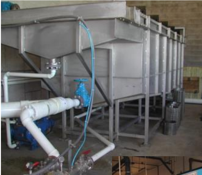
Dissolved Air Flotation
