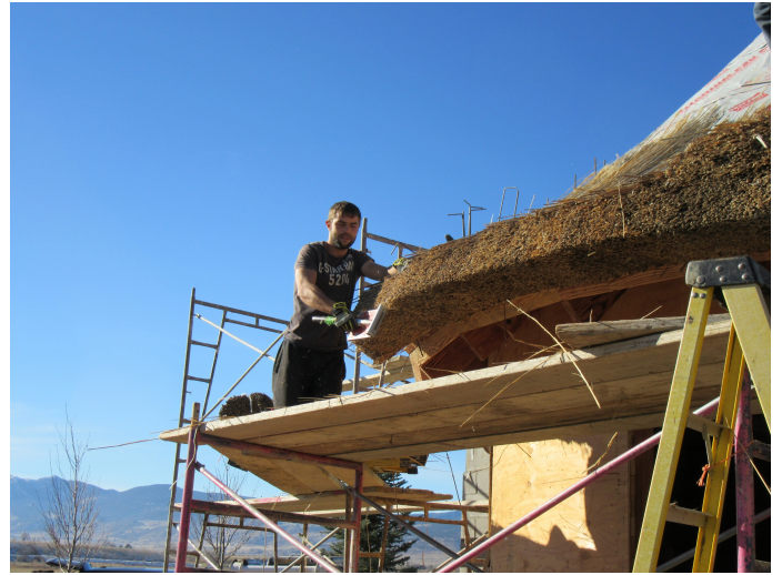
Using a leggett to 'dress' each course upon completion.
