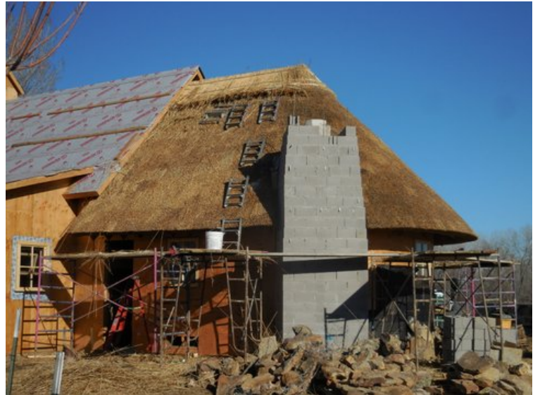
Using a leggett to 'dress' each course upon completion.
