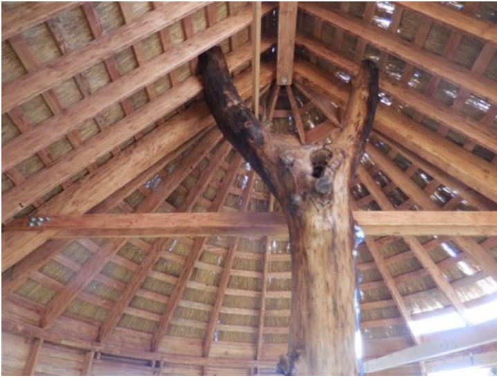
Interior view during installation of first layer of thatch.
