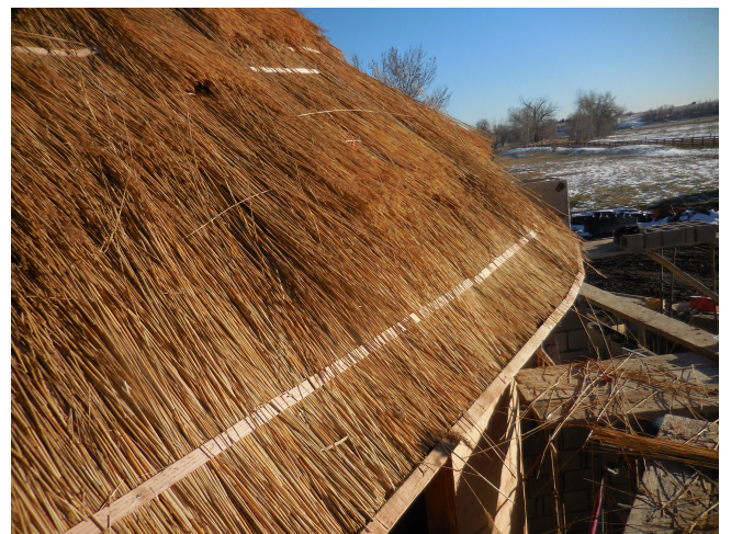
Bundles of reed through installation process over both purlins and solid decking. Hooks & sways (steel rods) are being used by Thatcher McGhee.
