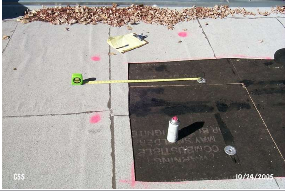
Fastener position and count is important
