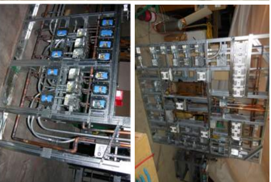
Medgas pipes and MEP rough-in
