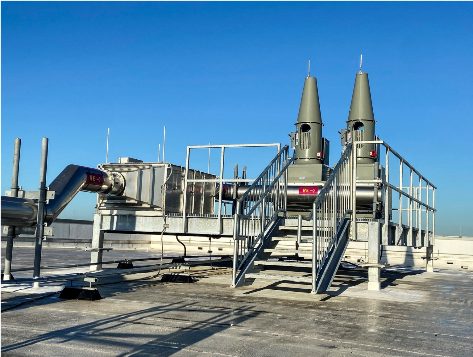
Figure 12: 4SCR4 Radioisotope fans, filter, and platform
