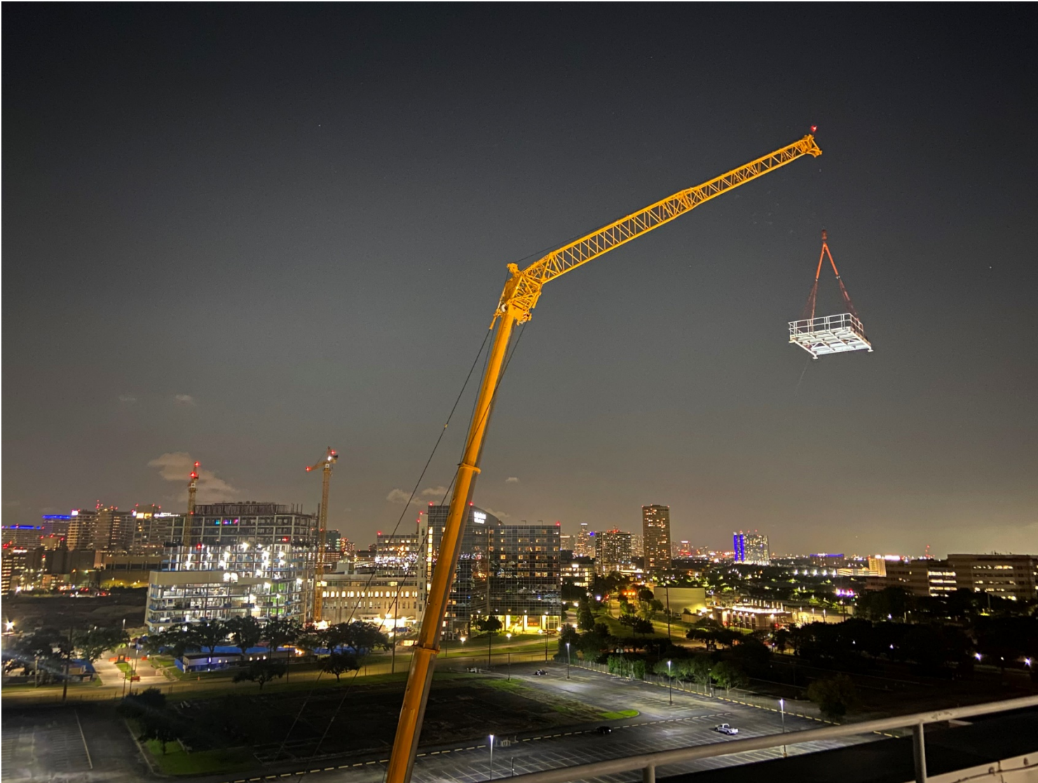
Figure 13: 4SCR4 Platform Crane Lift
