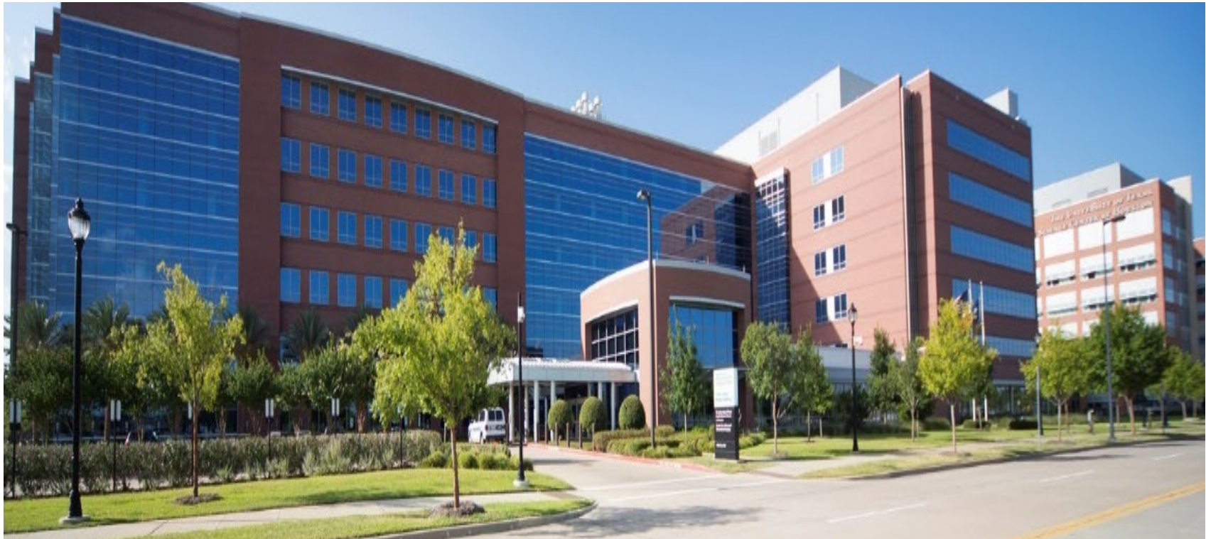
Figure 4: South Campus Research buildings 3/4
