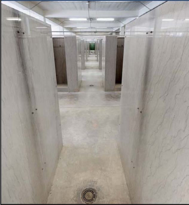
THE UNIVERSITY OF TEXAS AT AUSTIN | ANNA HISS GYMNASIUM | LEVEL 1 BEFORE AND AFTER
