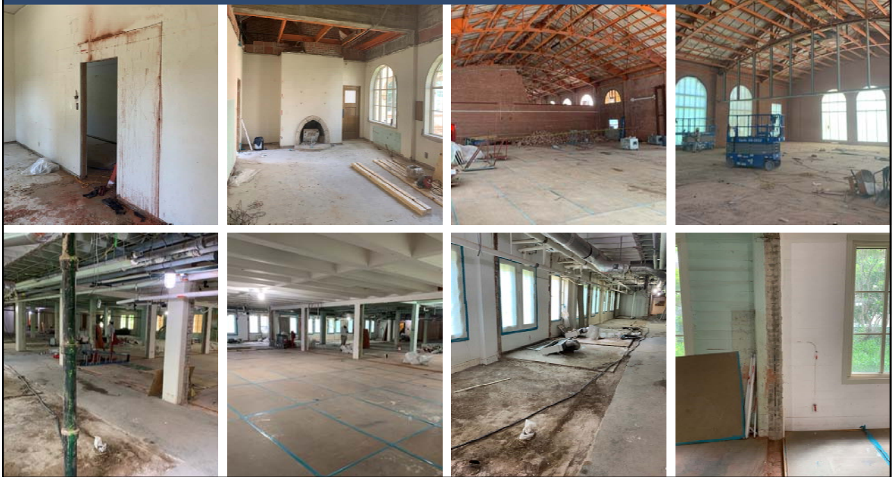
THE UNIVERSITY OF TEXAS AT AUSTIN | ANNA HISS GYMNASIUM | CONSTRUCTION PHOTOS
