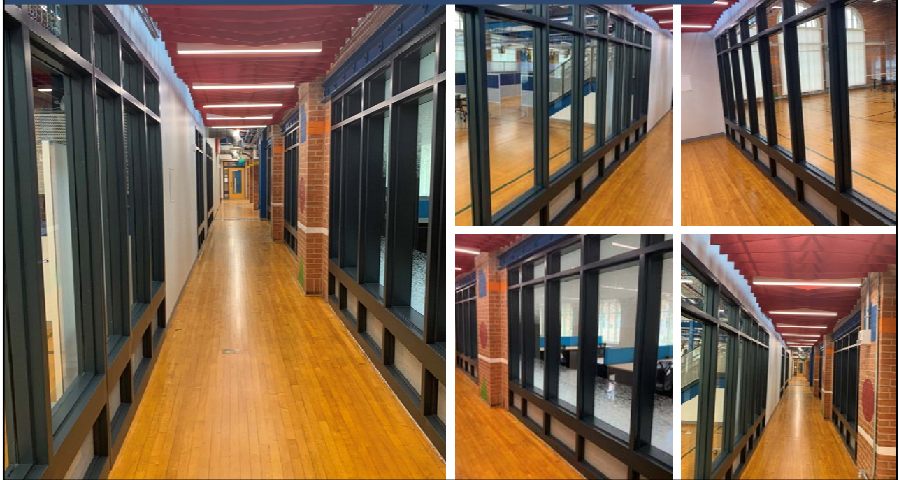
THE UNIVERSITY OF TEXAS AT AUSTIN | ANNA HISS GYMNASIUM | LEVEL 2 SOUTH WING CORRIDOR
