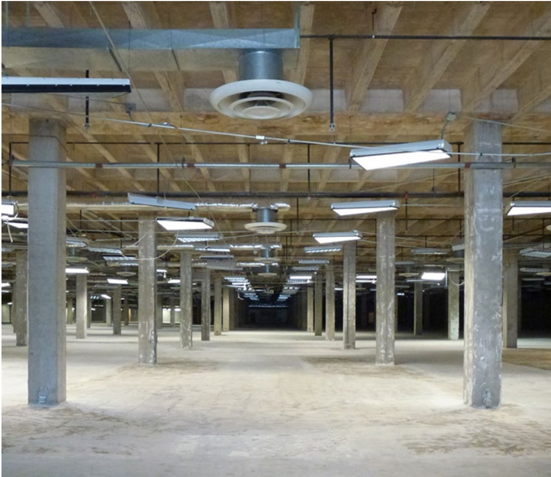
Highland Phase I BEFORE
