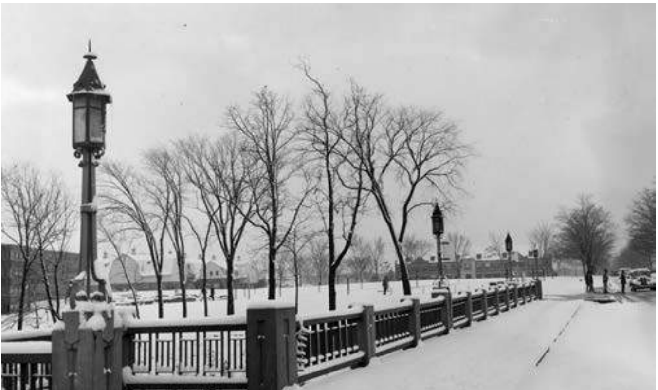
Rebuilt 1936-Era Bridge from 1951
