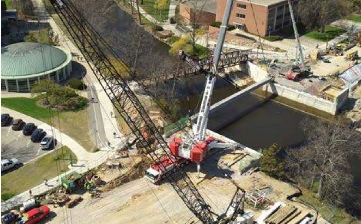
Steel beams being installed
