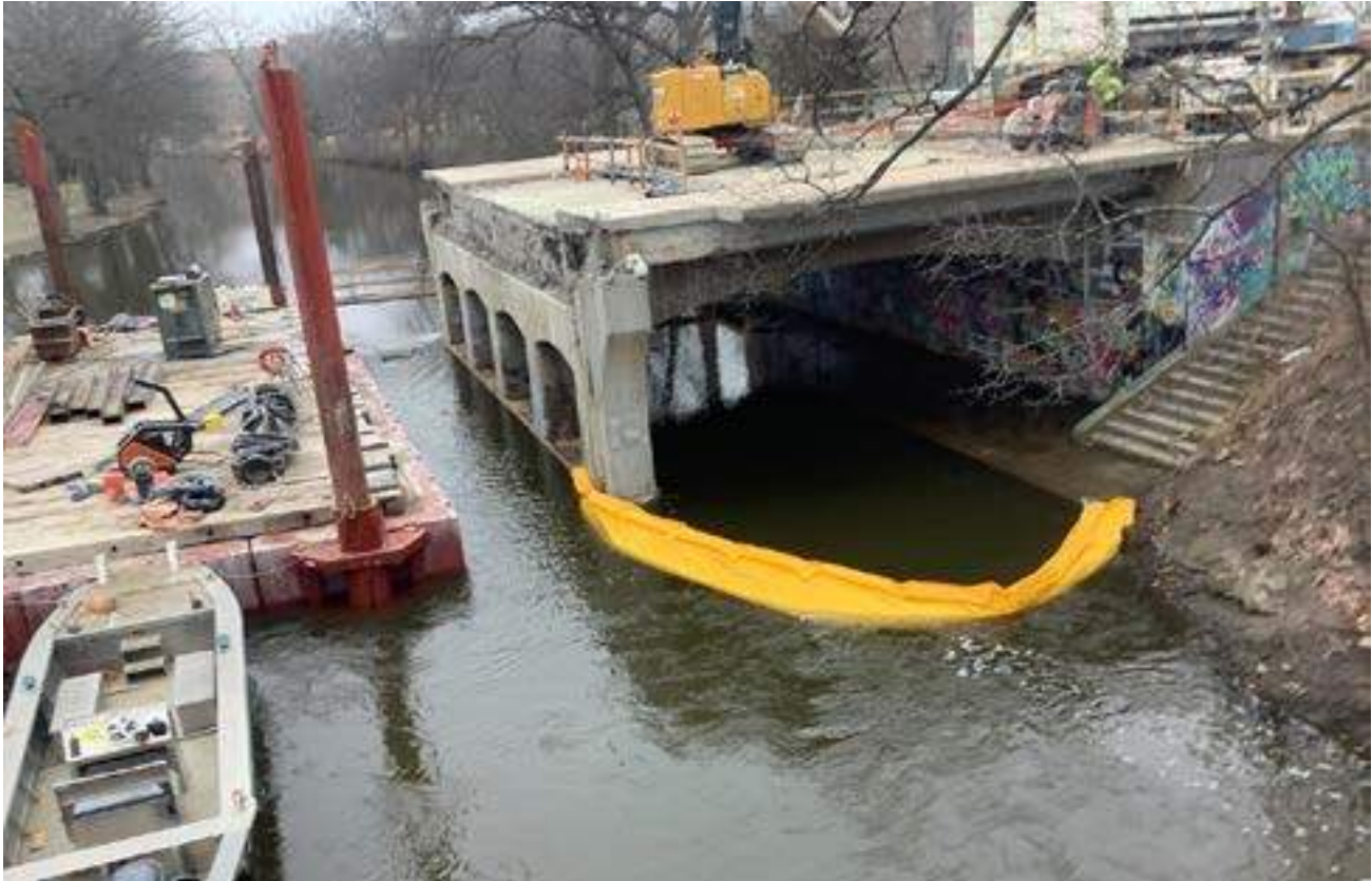
Barge used during demo for worker safety and in-river turbidity curtain for water protection
