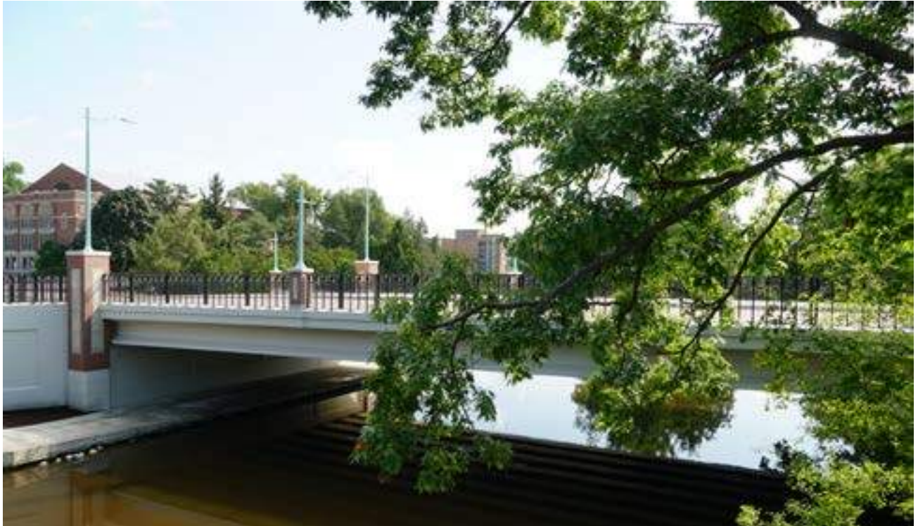
The new vehicular bridge also served as a critical utility corridor.
