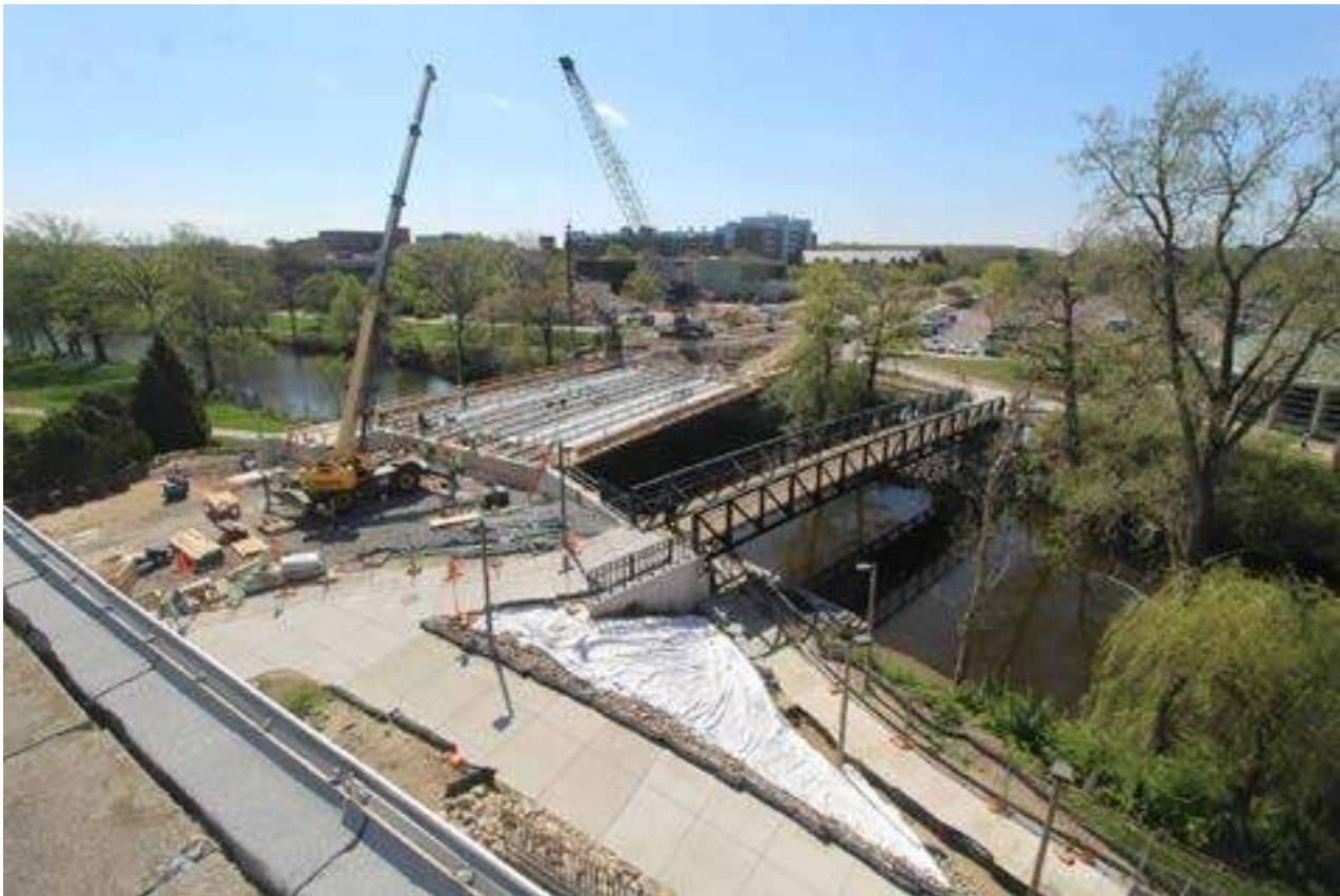
Setting Steam and Condensate
