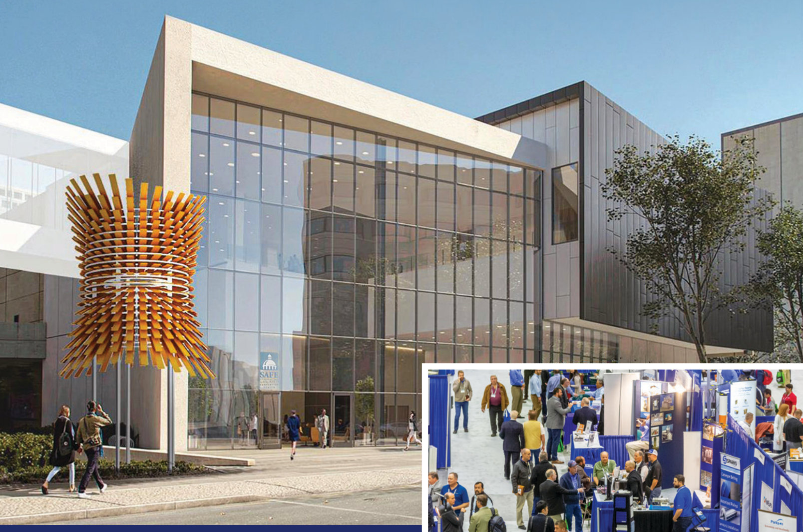
The newly renovated Sacramento Convention Center has been renamed the SAFE Credit Union Convention Center.
