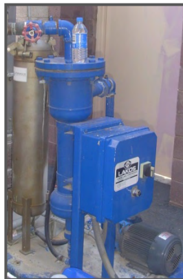
Figure 7.68 - Cyclone Separator with Bag Filter
