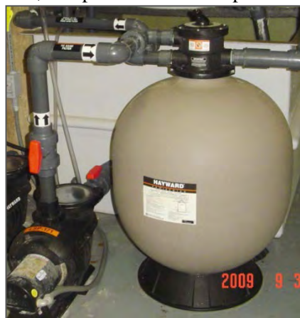
Figure 7.66 - Typical Sand Filter
