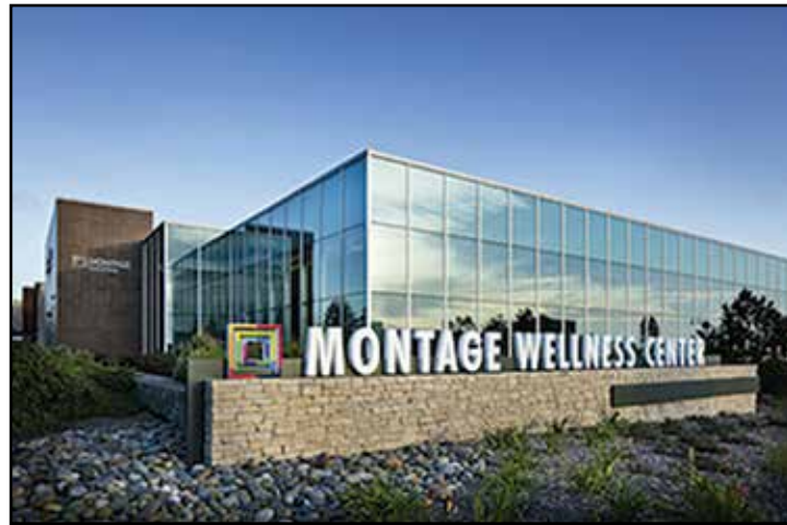
New 800 sq. ft. facility in Marina donated by Montage/CHOMP Foundation
