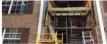
Exterior & Staircase Repairs
