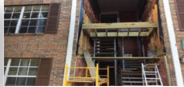
Exterior & Staircase Repairs
