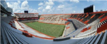
Pressure Washing / Gators Stadium
