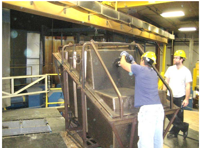
5.1.5 Pack vent tube and install the vent with the hook and utility wire.
