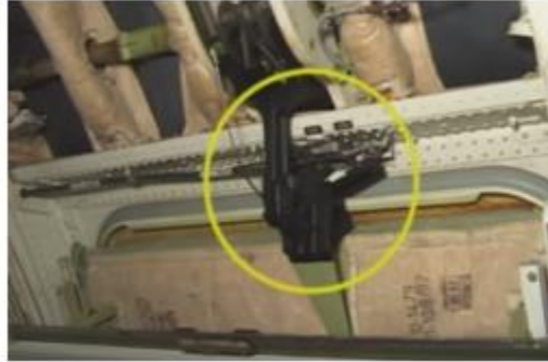
Figure 400: Entry/Service Door Ground Lock Pin.
