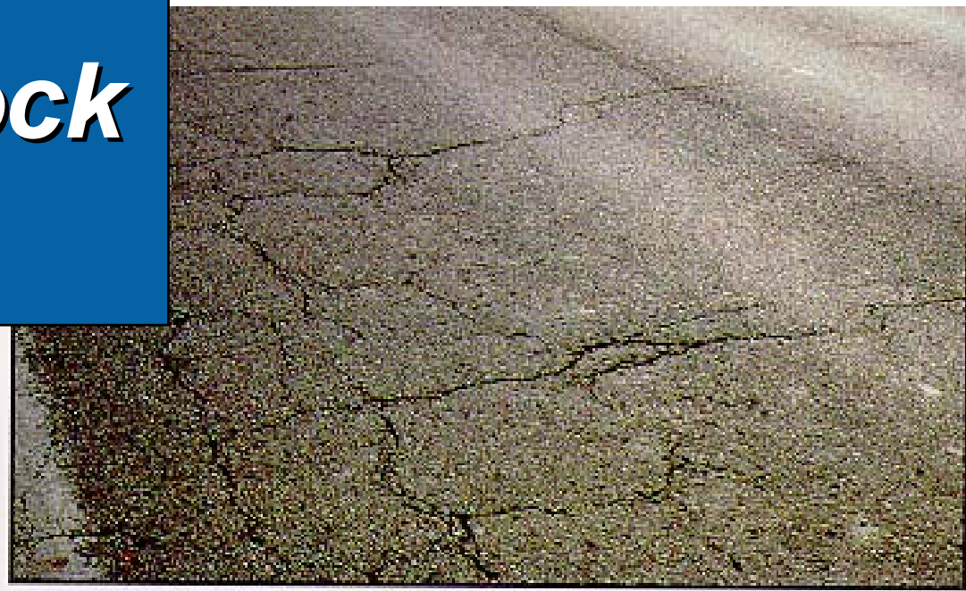
FIGURE 10 ACP 2. High Severity Block Cracking
