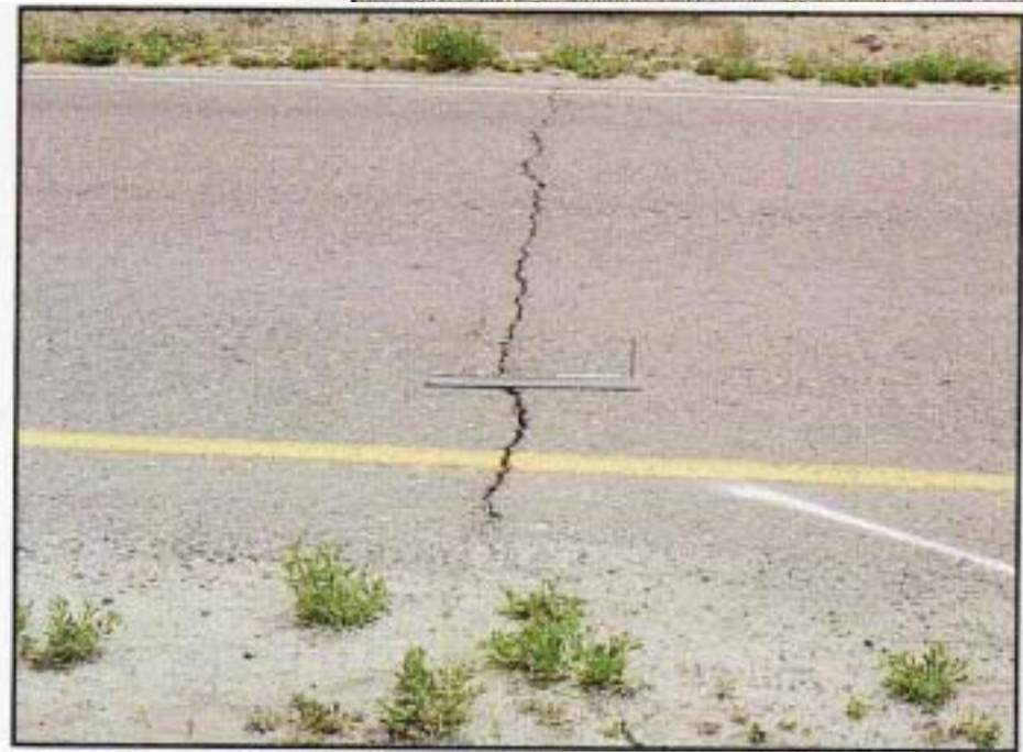
FIGURE 21 ACP 6. High Severity Transverse Cracking
