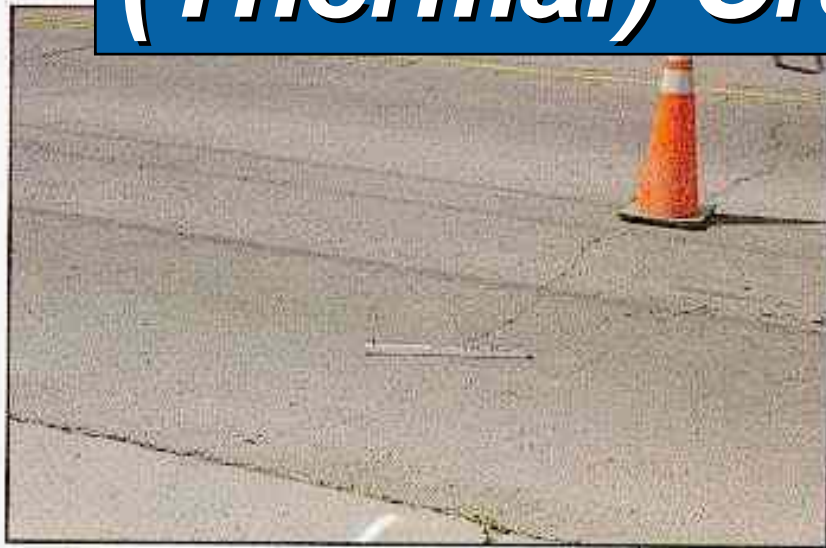
FIGURE 20 ACP 6. Moderate Severity Transverse Cracking
