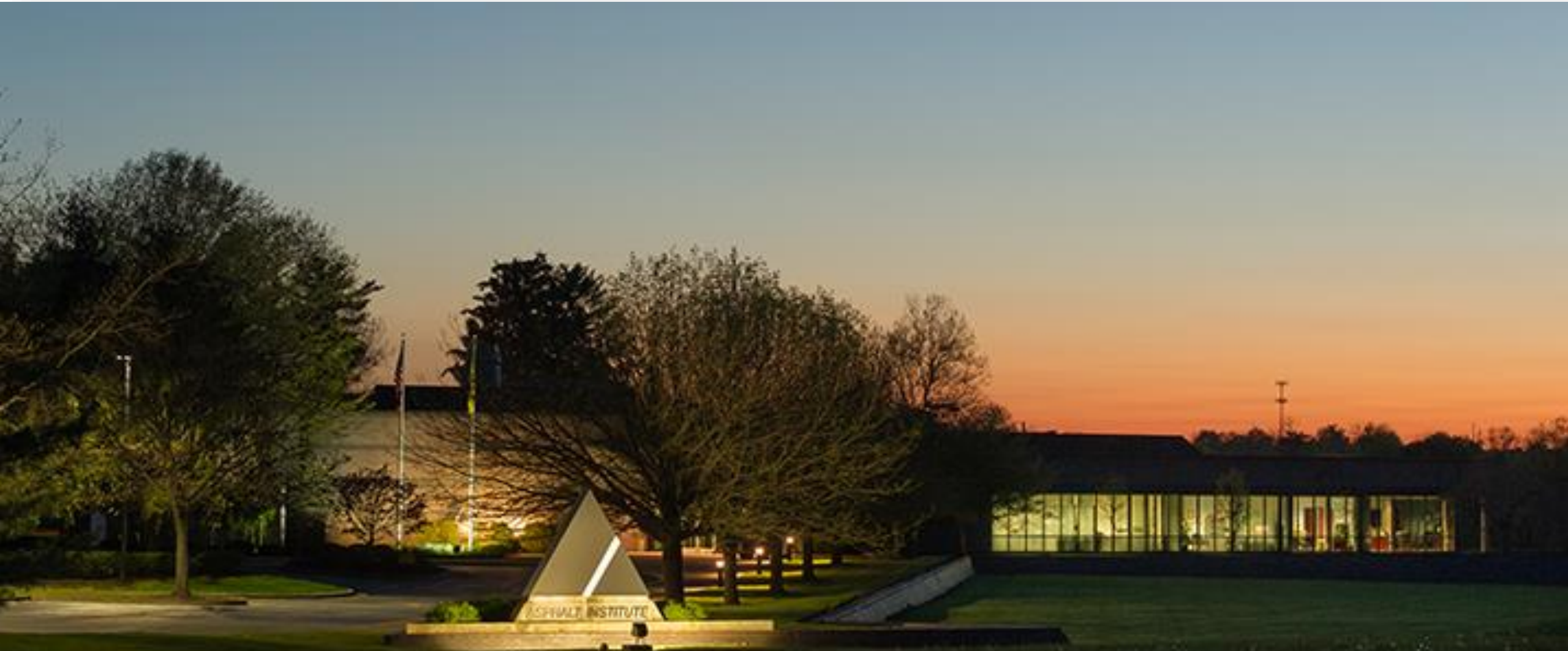
Asphalt Institute Lab & HQs, Lexington, Kentucky
