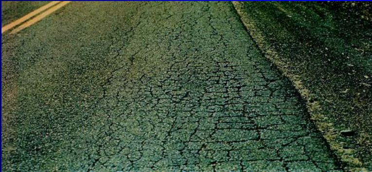
Fatigue (Alligator) Cracking
