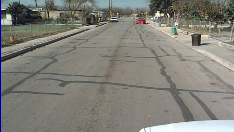
Crack Seal Application
