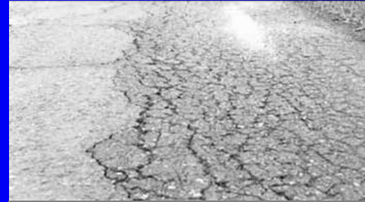
Alligator cracking
