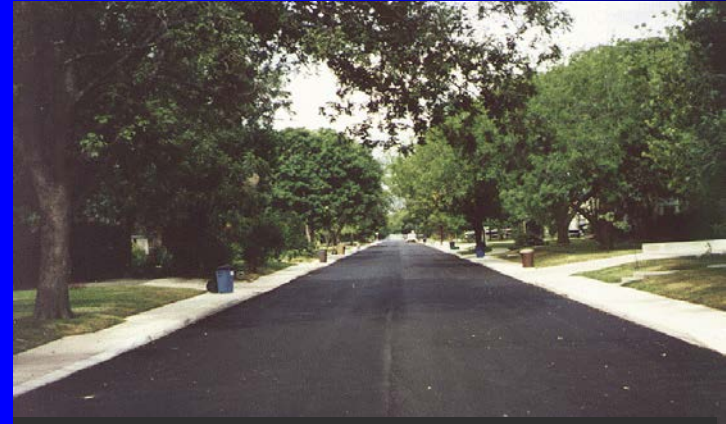
Slurry Seal Application
