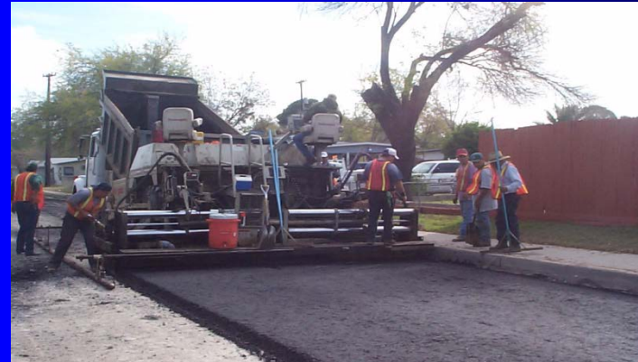
Asphalt Overlay
