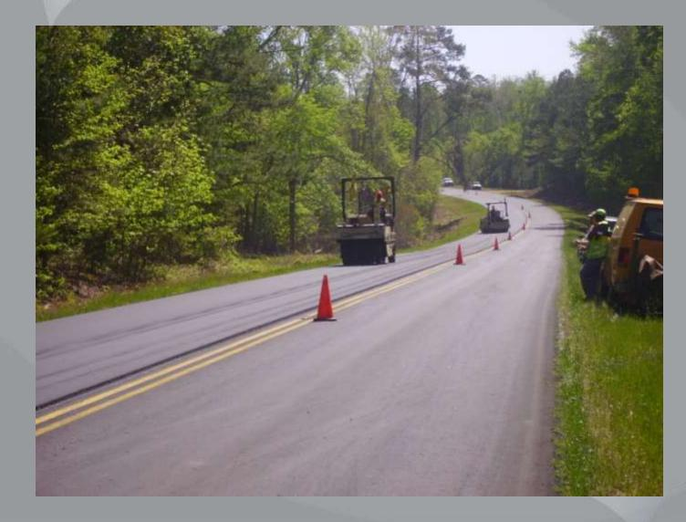
Superpave 9.5 mm Crumb Rubber Mix Design >AC content ...... 5.6%
