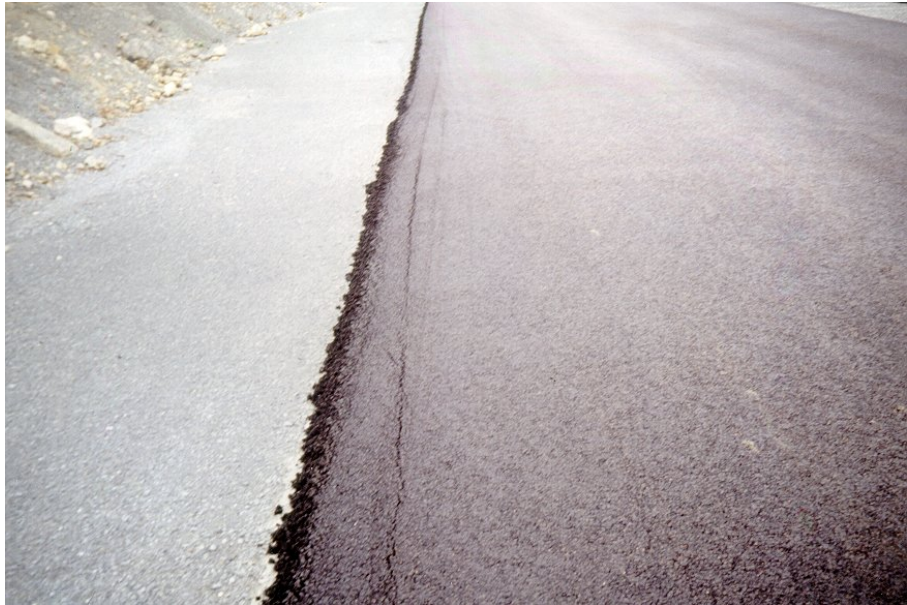
15 t tandem vibratory roller 8 passes
