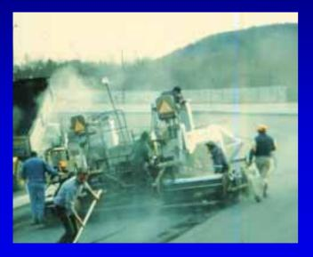
**EXAMPLE - PG 70-22** Lab Mix Temp: 333°F -343°F DOT allowed contractor to select mix temp > Target +/- 25°F Contractor selected Job Mix Range: 345°F - 395°F Temperature Lowered to 315°F - Improved Density and Ride
