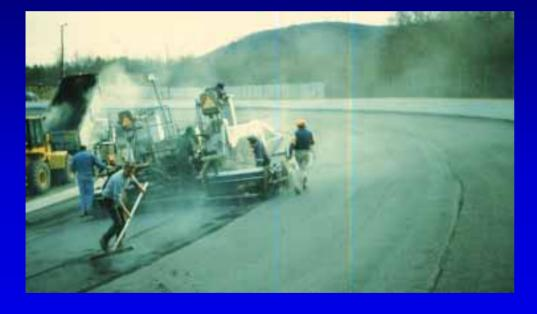
Superpave – new technology indirectly led to problems Emission episodes around the country Asphalt fumes are an irritant - worker
