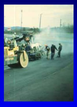
Excessive aging during construction Excessive fumes Tender mix Asphalt drain-down -**SMA and OGFC** mixes
