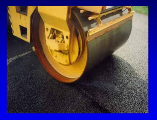
SUPERPAVE coarse mixes may be hard to compact Poor density may mean permeability -**FL** experience DOTs are focused on density Contractors are focused on density
