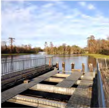
Pre-existing weir with failing maintenance deck
