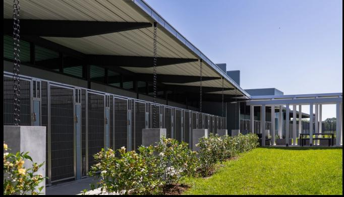
**CLERESTORY WINDOWS IN THE DOG DORMS** ALLOW FOR NATURAL LIGHT TO FLOOD THE INTERIOR WITHOUT GLARE AND HEAT GAIN. AN EXPOSED PERFORATED STRUCTURAL METAL DECK WITH ACOUSTICAL **INSULATION HELPS DAMPEN** SOUND IN THE SPACE. A "BARK WALL" SEPARATING EACH ROW OF DOG RUNS KEEPS THE DOGS FROM SEEING EACH OTHER AND MINIMIZES BARKING, A SPECIALLY DESIGNED HVAC SYSTEM ALLOWS FOR AMPLE AIR CHANGES TO MINIMIZE UNPLEASANT SMELLS.
