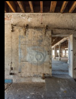
Historic Sliding Fire Door (2016)
