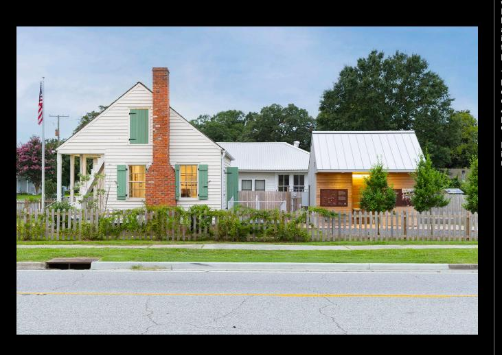
The site is enclosed with a wooden picket fence made of cypress, a wood native to South Louisiana. Pickets are widely spaced both to lighten the sense of enclosure and also to provide security by introducing a porous barrier rather than an opaque one which would provide a hiding place.
