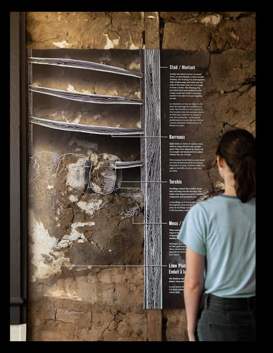
The building itself functions as an exhibit: Exposed areas of bousillage construction are overlaid with explanatory graphics, showcasing the technology and history behind the architecture.
