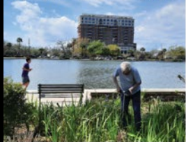
Groundwater Monitoring System Installation
