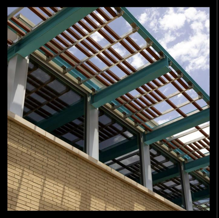
The brise-soleil's terracotta baguettes are mounted between extruded anodized aluminum tracks, which are in turn suspended from the primary structure, a turquoise-painted steel frame. The color selection for the steel references turquoise beads encountered among the tribe's archaeological record. Turquoise beads have cultural significance not only for this tribe but also for Native communities across the Americas.
